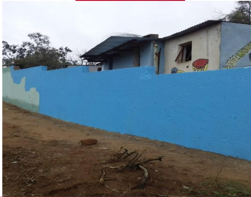
Painting of the wall in progress
