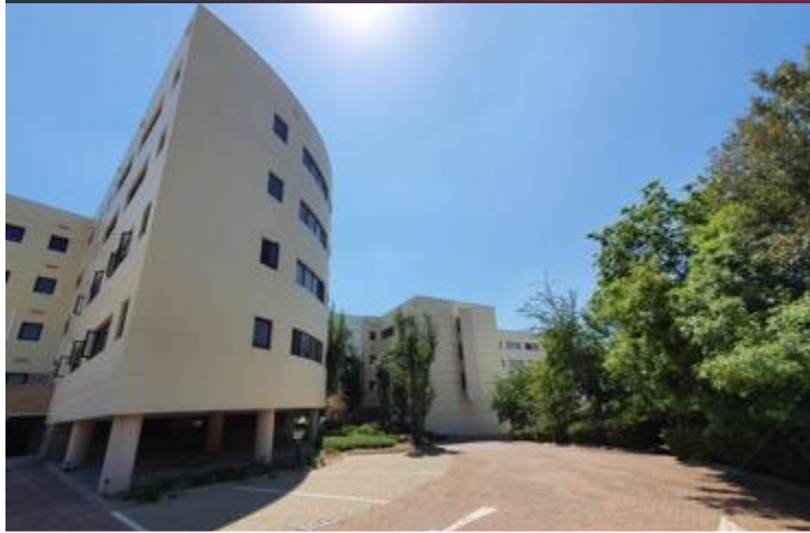
IBG revamped into Midrand Gate
