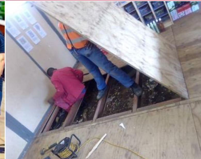
Repairs to the loose flooring
