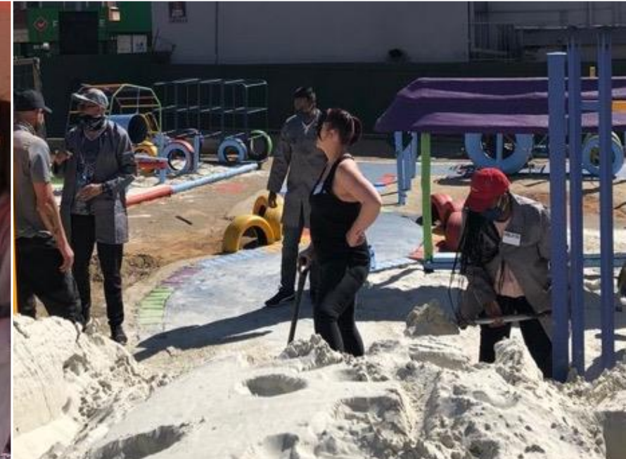
Filling the playground with safe-sand
